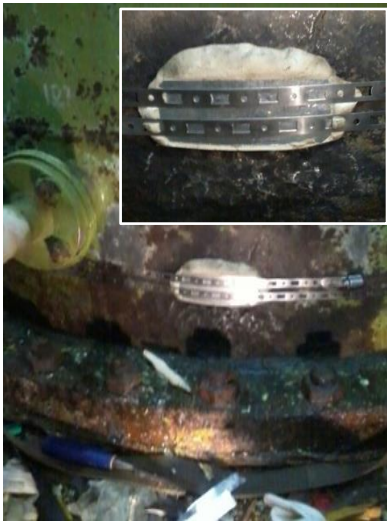
SealXpert™ stainless steel clips and Seal Stic™ was applied onto the pipe to arrest leak
