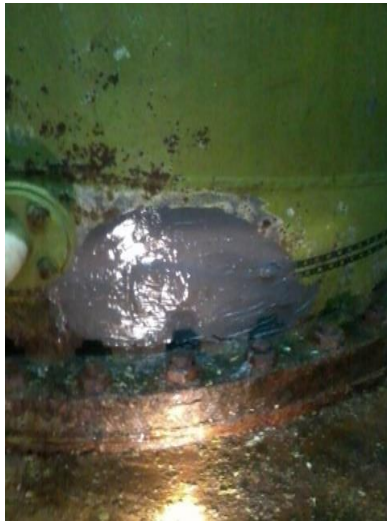
SealXpert™ Repair Putty was applied onto the affected area
