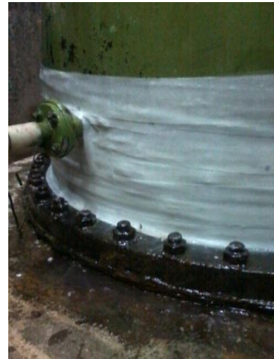
Wrap Seal PLUS™ Fiberglass Tape was applied for pipe reinforcement
