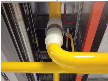
Pipe thinning and crack on pipe elbow
