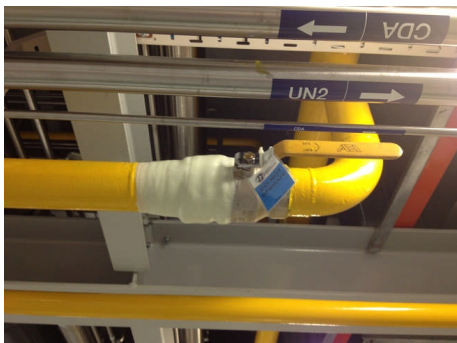
Applying SealXpert™ repair putty
